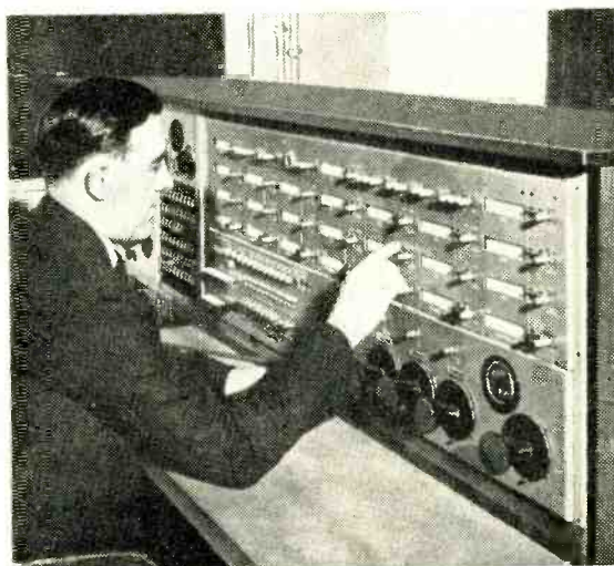
AUTOMATIC SWITCHING. Sound broadcast programmes for the B.B.C.'s West Region transmitters are switched to their destinations by a system something like an automatic telephone exchange. It is operated by a single engineer at this control desk, which is the "nerve centre" of a new control room recently installed at the West Region headquarters in Bristol.
